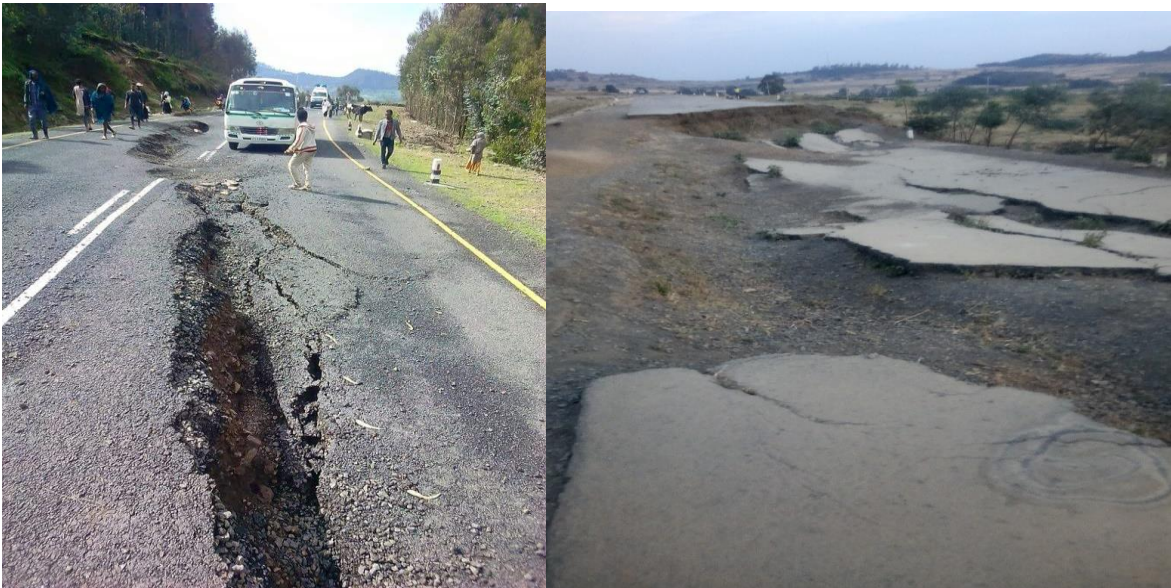
Figure 7: Drainage Problems (Road failure due to scouring of water) (Injibar – Dangila road section)
