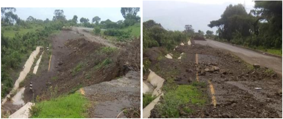
Figure 4: Sinkhole failure of the road due to scouring of water in the road segments
