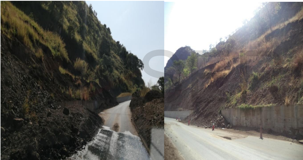
Figure 4: Sinkhole failure of the road due to scouring of water in the road segments
