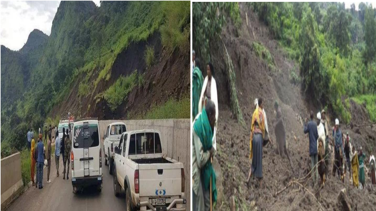
Figure 14 : Model 4- road failures due to instability of slope presentation diagram & images
