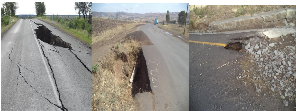
Figure 3: compressibility of soil/settlement problem
