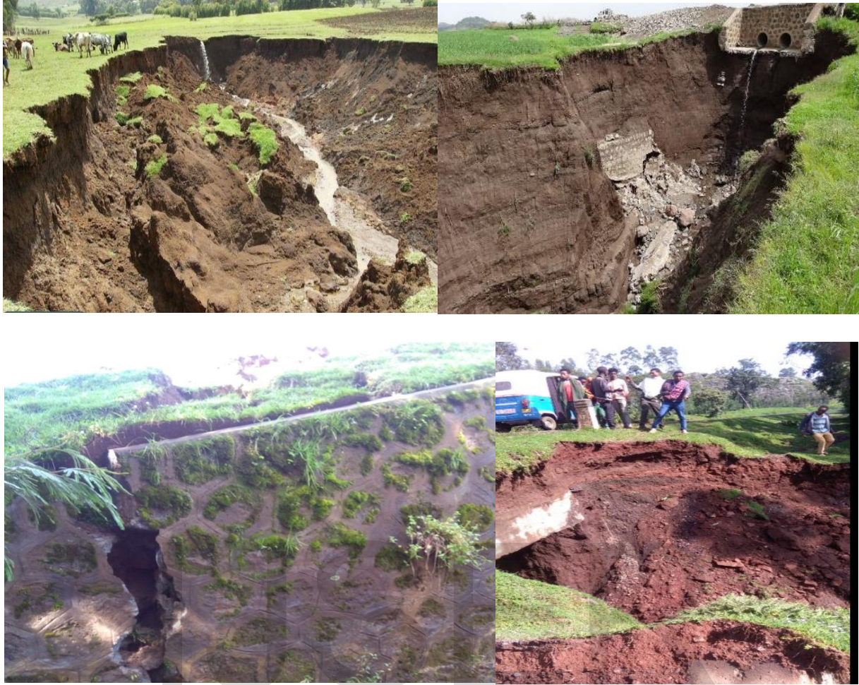
Figure 7: Drainage Problems (Road failure due to scouring of water) (Injibar – Dangila road section)
